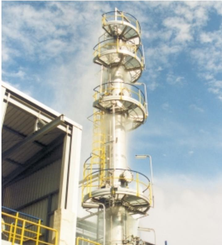
*On high reaction columns, nozzle rings must be used to position the water spray protection at several different heights.*
