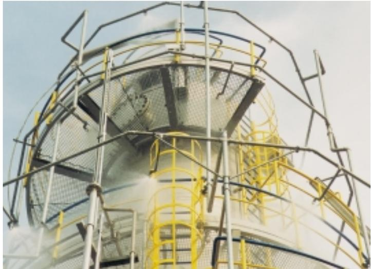
Since many of these fire gases are water-soluble, the substances are bonded and carried away in the extinguishing water. In this way, TOTAL WALTHER water spray extinguishing systems reduce corrosion damage and maintain the operating capability of your machinery and plant.
